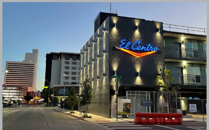
El Centro, Northern Nevada Community Housing Reno, Nevada
