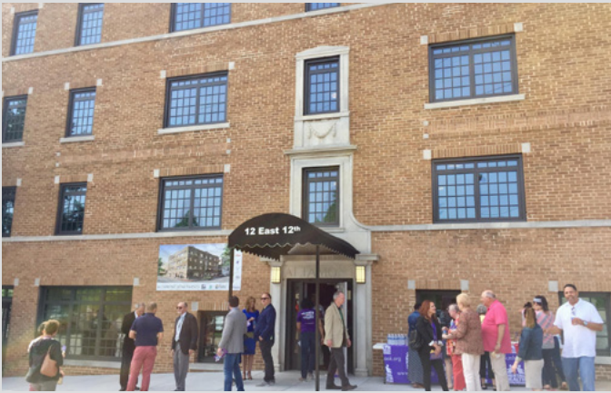
Altamont Apartments, Mental Health Association of Oklahoma PSH for homeless and chronically homeless people with disabilities Tulsa, Oklahoma
