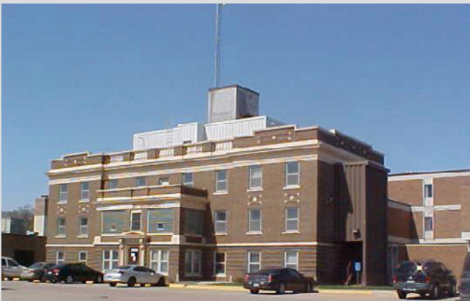
Former Boys' and Girls' Home converted to Family Resource Center affordable housing for seniors, Columbus Community Foundation and Mesner Development Columbus, Nebraska
